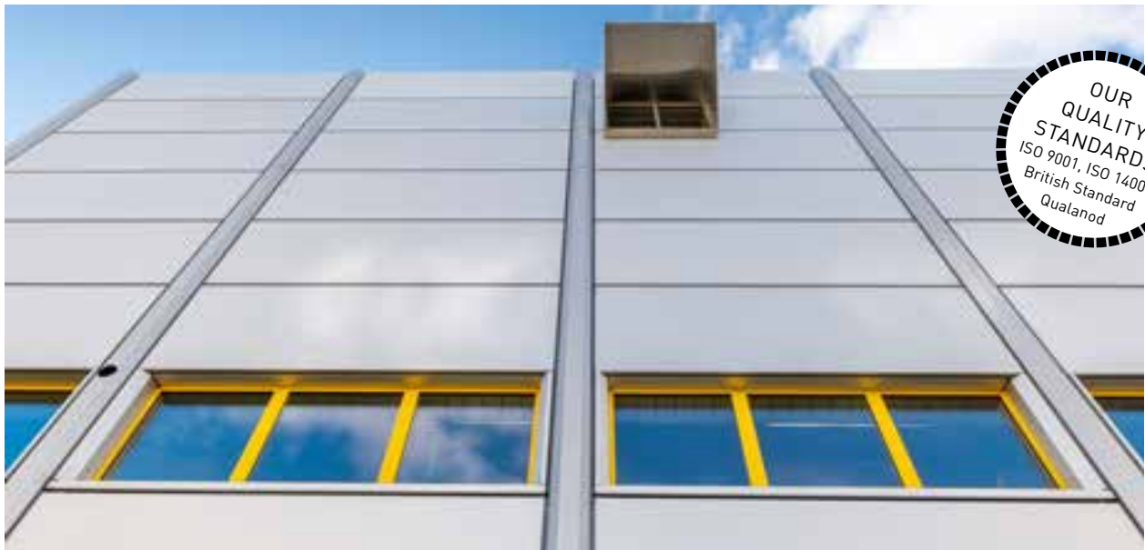
Freshly cleaned anodised façade
